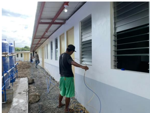
Electrical wire installation
