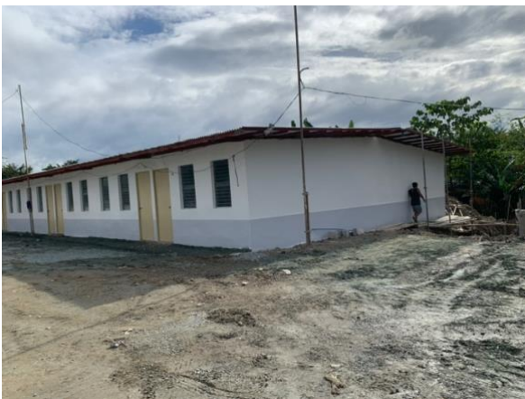
Transition houses (Rowhouse)
